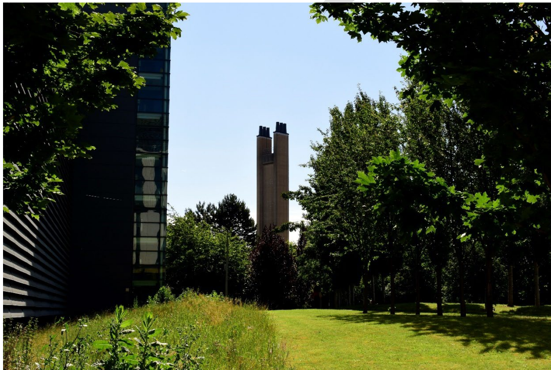
Image 5: Addenbrooke's Hospital incinerator chimney
